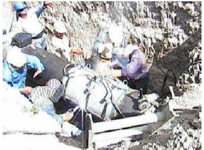
Figure 2: Compression Steel Sleeve Installation
