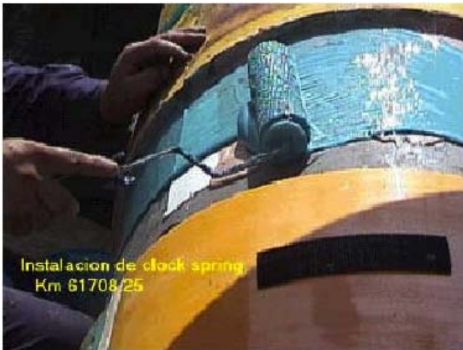
Figure 3: Composite Sleeve Installation
